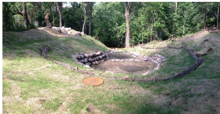
Figure 1. RL Stevenson School Ravine Restoration: After Restoration Photograph by D. Kalmon
